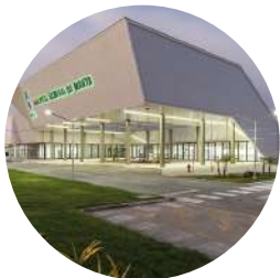
16 Hospital Manta ECUADOR
