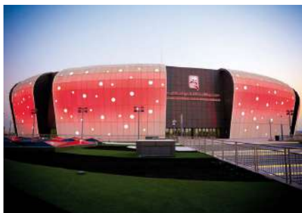
Qatar Handball Stadium illuminated with Square Grazer®
